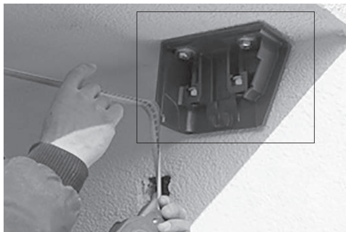
Fig. 07: Aligning brackets (ceiling installation here, for example)
